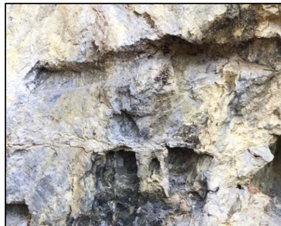
Figure 9. Blast scarring on the exterior cave wall near the entrance.
